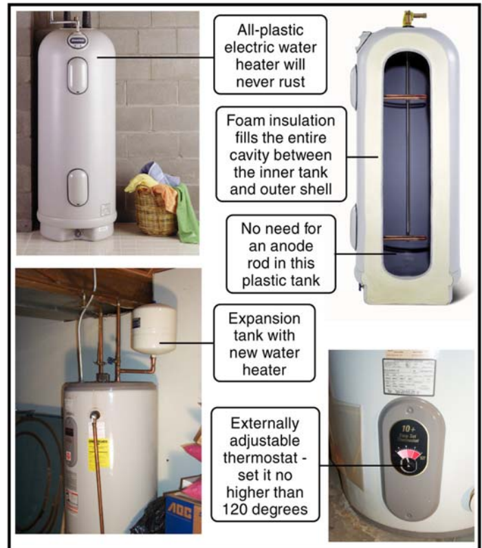
New water heaters save money, last longer
